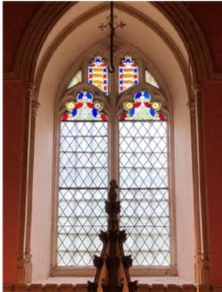
For the new panels, various tones of antique clear green mouth-blown restoration glass from Poland were chosen for the decorated sections. The inherent 'bottling', bubbles and defects of mouth-blown glass are always
